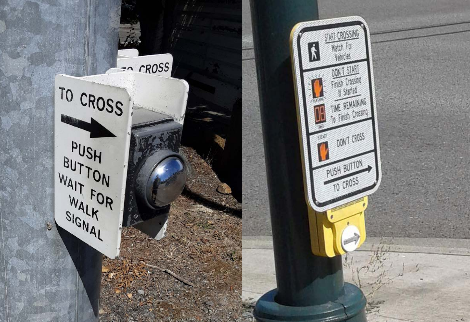
Figure 2-17 “H-style” (left) and APS-style pedestrian pushbutton (right)
